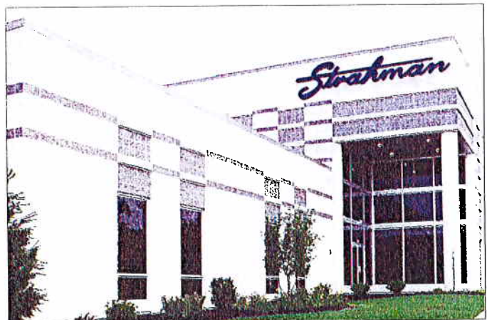
J.G. Petrucci has developed a 52,500-square-foot speculative facility within the Lehigh Valley Industrial Park VI for Strahman Valves.
