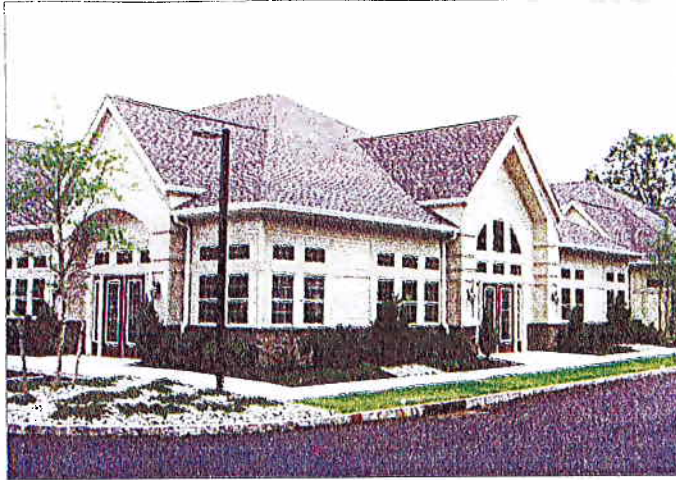
Larken Associates recently completed The Courtyard at Amwell, a 14,038-square-foot built-to-suit medical office space in Hillsborough, New Jersey.
