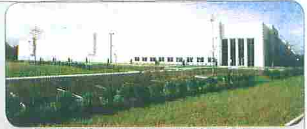
324 Half Acre Road, which has been sold to US Industrial REIT II
