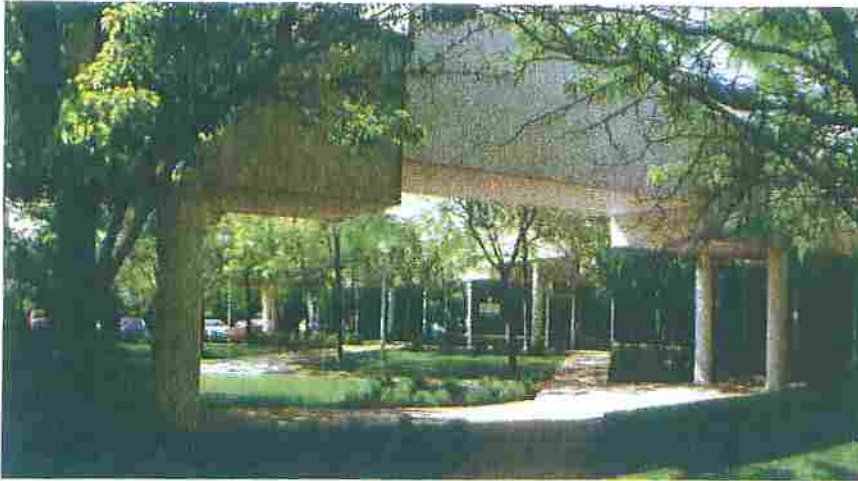
Eastman Companies' Regent Park, the 160,000 square-foot, five-building facility located on Route 10, Livingston. The office complex is situated in a landscaped park-like setting and offers a host of amenities including an on-site day care center and café, and 24-hour access.
