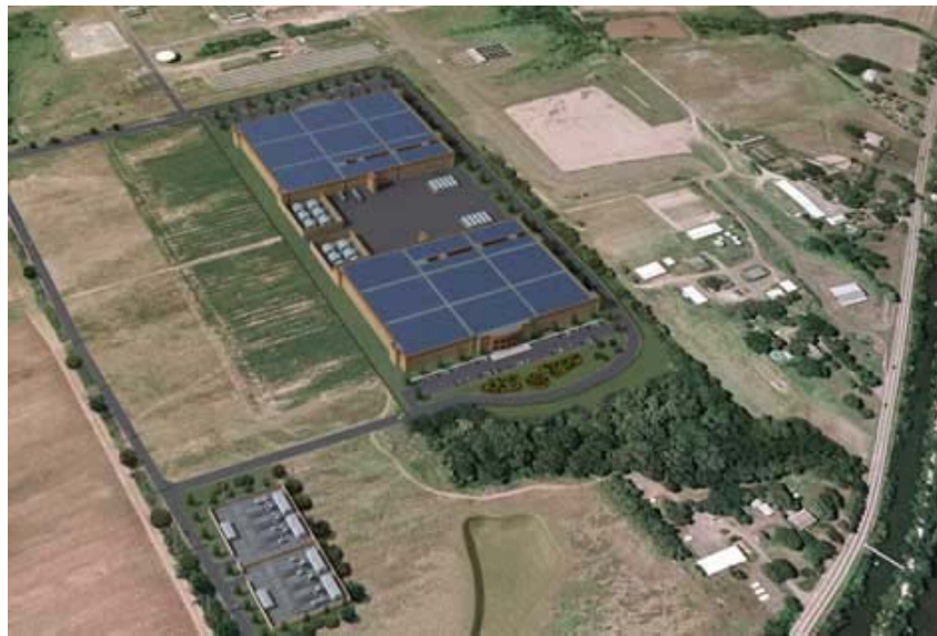
An aerial view of the site of the Somerset Technology Park, a new data center project from Russo Development in central New Jersey, including an illustration of a planned data center.
