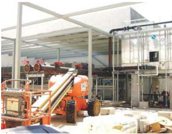
Photo: Gilbane Building
